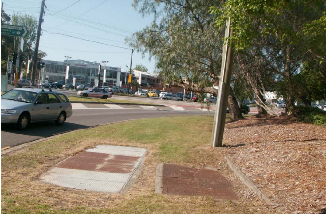
This is an adequate Clear Zone with the utility pole placed well away from the road.
