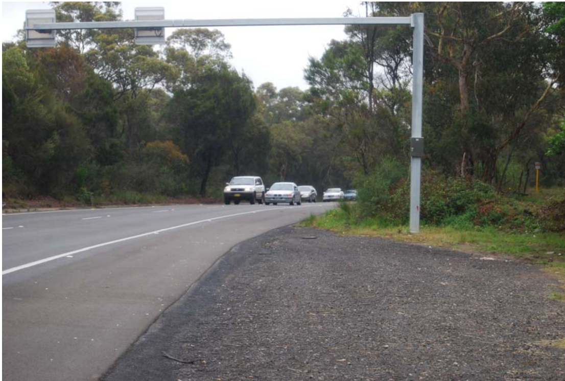
Signposting is installed well away from traffic - providing an adequate Clear Zone.
