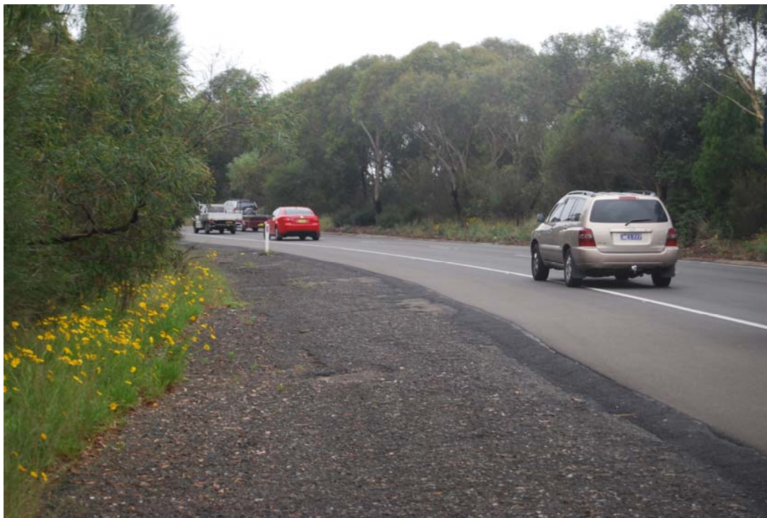
Providing an adequate Clear Zone on this bend reduces the potential of a vehicle colliding into a utility pole.
