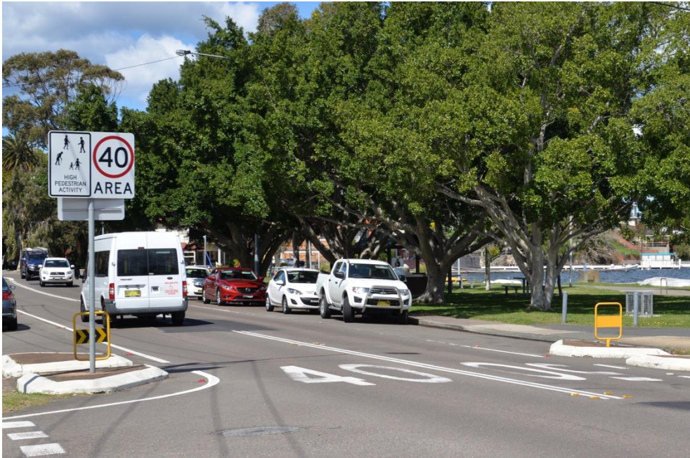
Figure 5: Belmont – Road narrowing using islands and linemarking
