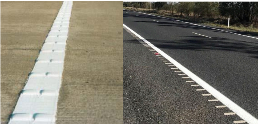
Figure 1: Examples of ATLM installed on top of an edge line (left) and adjacent to an edge line (right)
