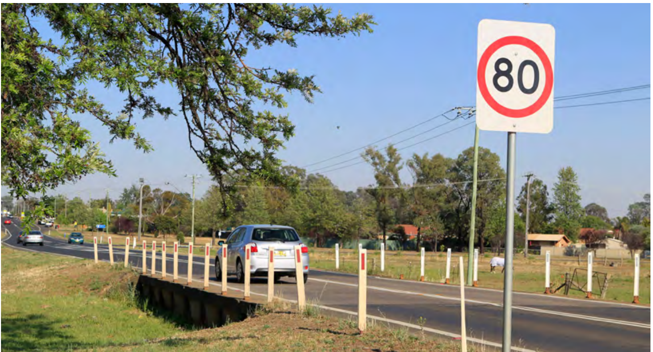
Photograph 2.2: A series of culverts over a flood prone area west Tamworth
