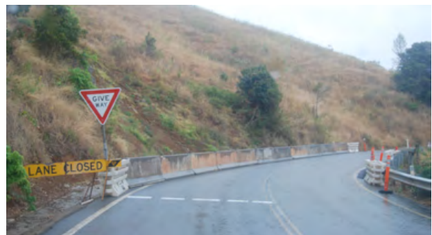
Photograph 2.8: A partial road closure following a land slide on eastern escarpment
