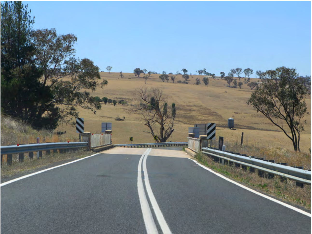
Photograph 2.9: Bridge over railway line near Woolbrook west of Walcha
