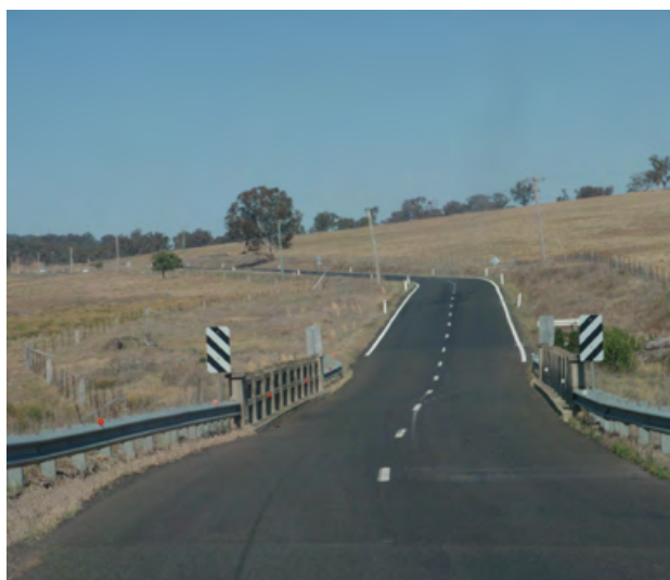
Photograph 1.6: Western approach to Chimney Swamp Creek west of Walcha
