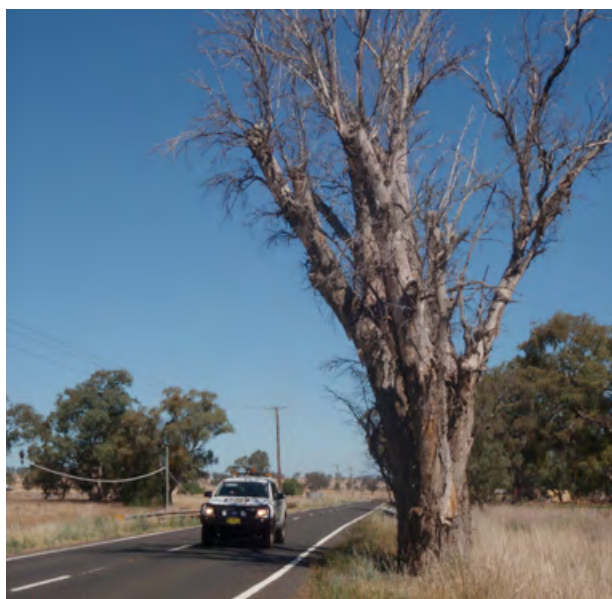
Photograph 2.6: A dead tree well within the clear zone west of Tamworth
