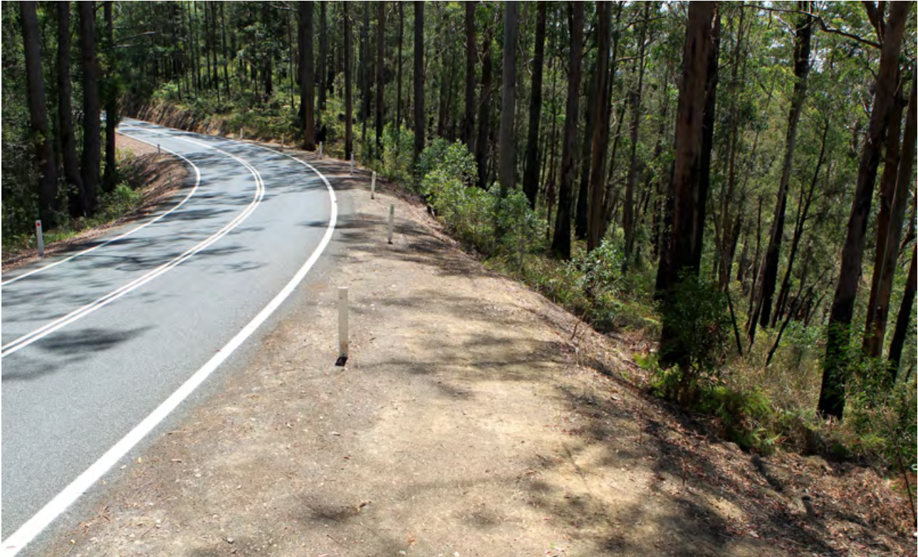
Photograph 2.7: Steep drop-offs and trees within the clear zone along the eastern escarpment
