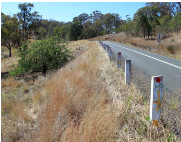
Photograph 2.5: Chain wire barrier west of Walcha
