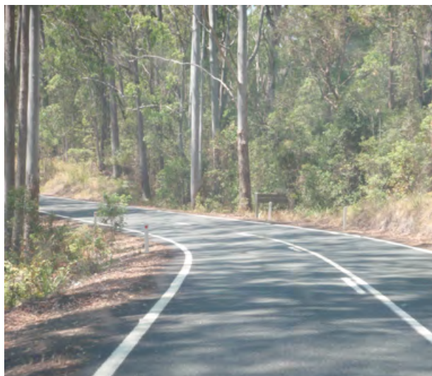
Photograph 1.7: Centreline marking permitting overtaking around curve
