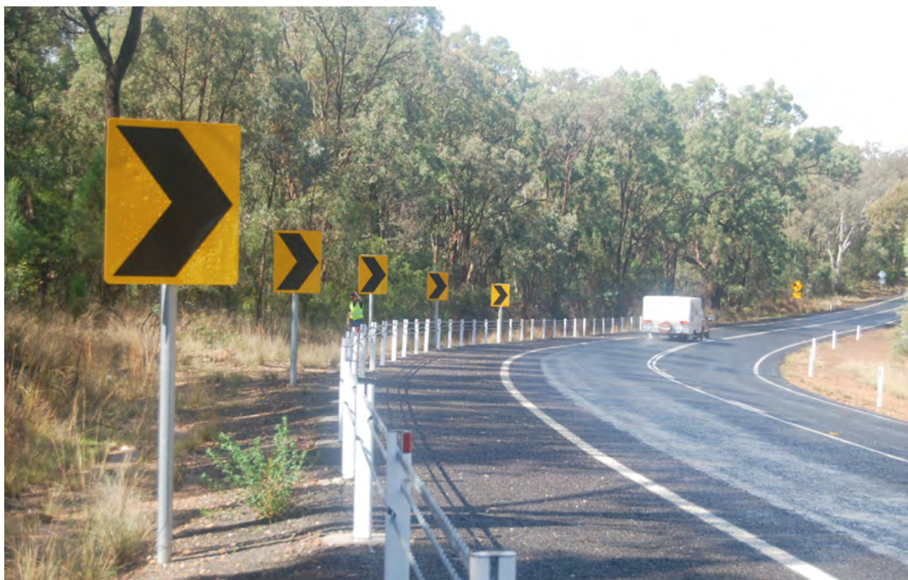
Photograph 2.10: Enhanced curve delineation east of Coonabarabran
