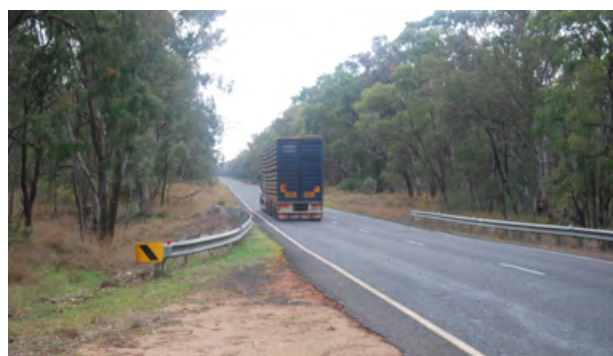
Photograph 3.11: A heavily timbered section of the road corridor east of Coonabarabran
