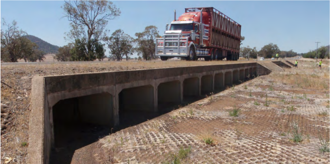
Photograph 3.3: Unprotected series of large culverts west of Gunnedah
